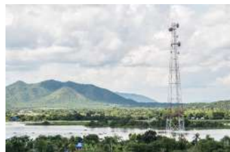
WIRELESS / BROADBAND / DATA CENTER Pg. 140
