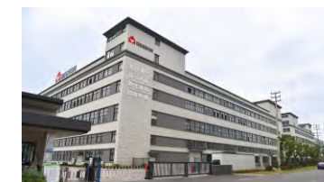
High-tech zone site
