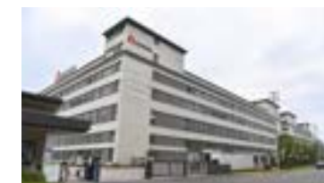
高新区工厂 High-tech zone site
